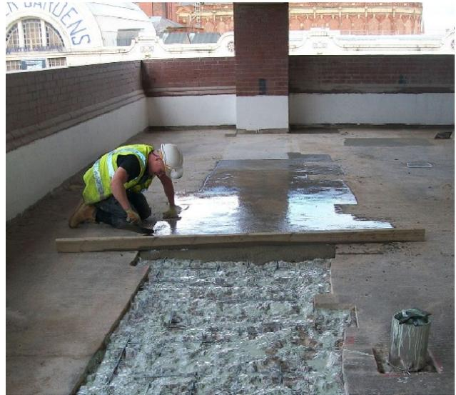
strength of 20 MPa at 2 hours, 50MPa at 24 hours and a drying shrinkage of <300 micro-strain at 7 days. The product shall be mixed, applied and cured in accordance with the manufacturer's written instructions to a correctly prepared substrate.
