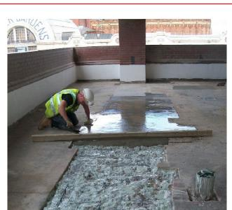
strength of 20 MPa at 2 hours, 50MPa at 24 hours and a drying shrinkage of <300 micro-strain at 7 days. The product shall be mixed, applied and cured in accordance with the manufacturer's written instructions to a correctly prepared substrate.
