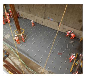
Where ground gas protection is required, Proofex Engage, in conjunction with Supercast Watertight Concrete, has been independently assessed as providing a protection score of 4.5 points, sufficient for all building types constructed in ground with a Characteristic Situation 3 hazard potential.
