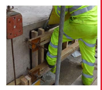
applied in sections generally up to 200 mm thick although greater thicknesses may be achievable dependent on the configuration of the repair location and the volume of exposed reinforcing steel. Consult the local Fosroc office for further information.
