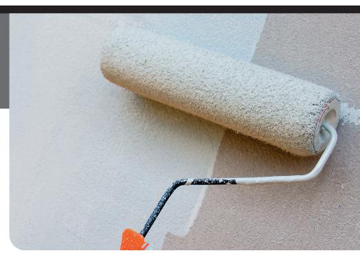
**Thermaldry Anti-Condensation Coating** is both thermally insulating and water repelling. It increases the wall temperature, thus reducing the 'dew point', or the temperature at which condensation occurs.
