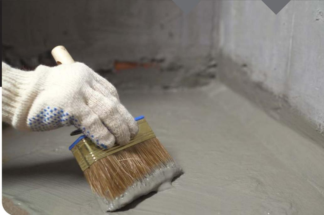
SBR Latex is a styrene butadiene copolymer latex, specially modified to be compatible with cement based mixes including ordinary portland cement or high aluminium cement. It may be incorporated into cementitious renders, screeds or patching mixes
